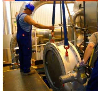
Installation of technological equipment
