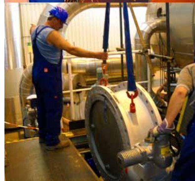
Installation of technological equipment
